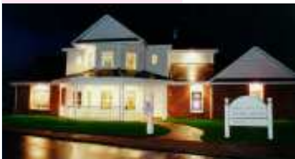
German home near Bremen built with a Timber Truss panelized package.
